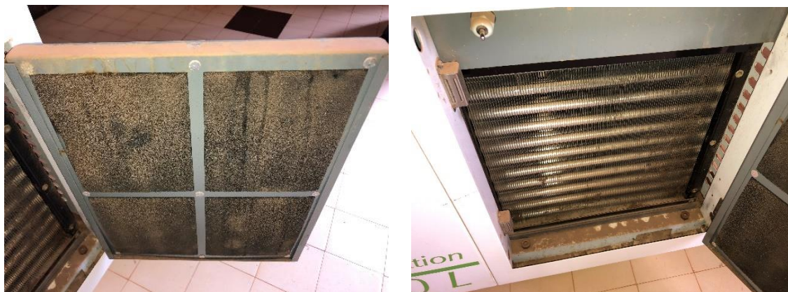
Figure 14 (a & b). Dirty filters found in non-working freezers.
