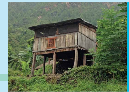
Completed goat shelter made from salvaged materials in Gorkha. Photo by CRS Staff
