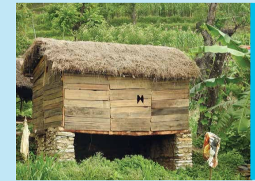
Completed goat shelter with a traditional thatched roof in Gorkha. Photo by CRS Staff
