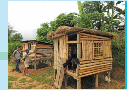
Completed goat shelters made using locally available bamboos in Gorkha. Photo by CRS Staff
