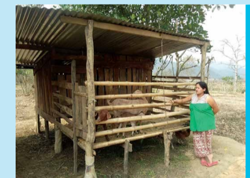
Completed goat shelter with corrugated galvanized sheet roofing. Photo by CRS Staff
